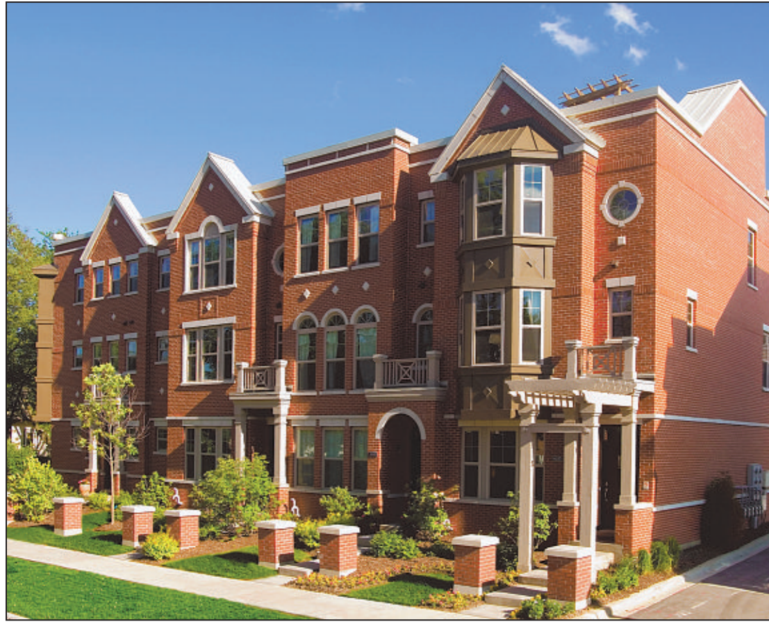
The Crossings at Morton Grove features red brick buildings adorned with limestone accents, wrought iron detail and individual arched brick entries.
